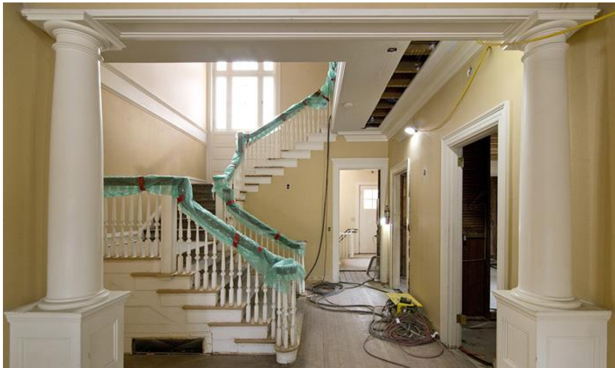
A 7,500-square-foot building in Northwest Portland built in 1892 as a home for a Portland physician is being renovated for Sloy, Dahl & Holst Inc. (Sam Tenney/DJC)
